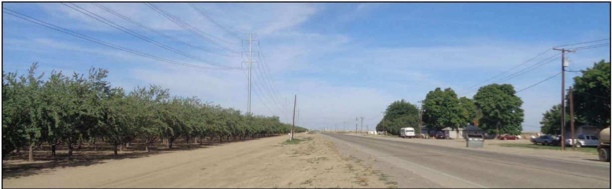
Photo 4: 230-kV Gen-Tie Monopole Line with Residences Opposite
