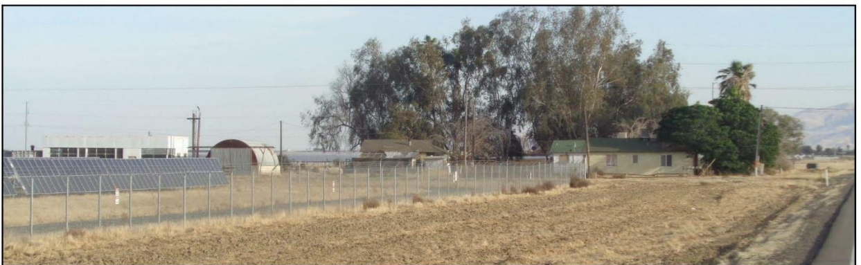
Photo 9: Solar Array with Adjacent Residence
